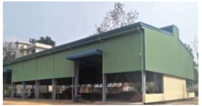
Multipurpose Shed at Jalalabad Cantonment Public School & College
