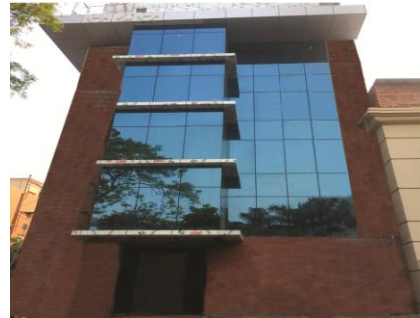
Admin Building, Acme
