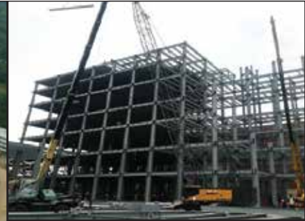
8-Storeyed Steel Structure for ACI Ltd Narayanganj.
