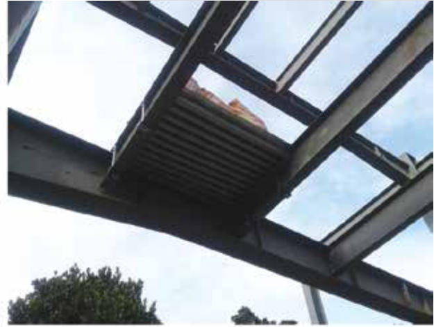
(b) At overhead floor level
