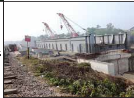
24 Nos Steel Railway Bridge, Laksham Akhaura.
