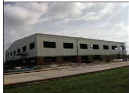
Factory Building, ISHO Ltd. Gazipur.
