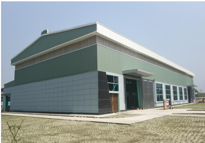
BMTF GALVANIZED SHOP
