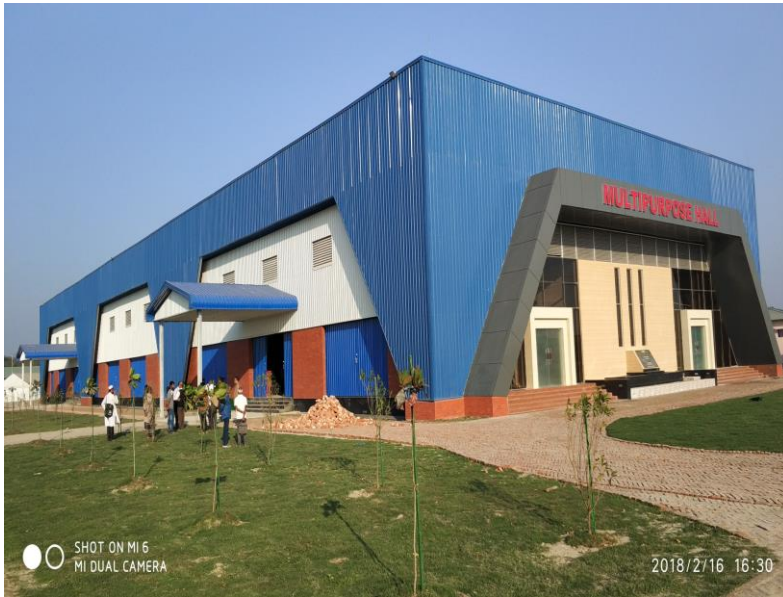
LEBUKHALI CANTONMENT MULTIPURPOSE SHED
